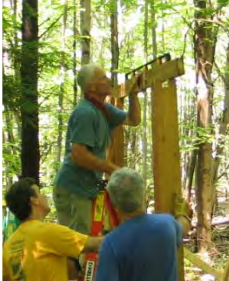
Aligning the tops of the legs (left) and squaring the legs using the MDO panel (right)
