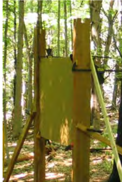
Aligning the tops of the legs (left) and squaring the legs using the MDO panel (right)
